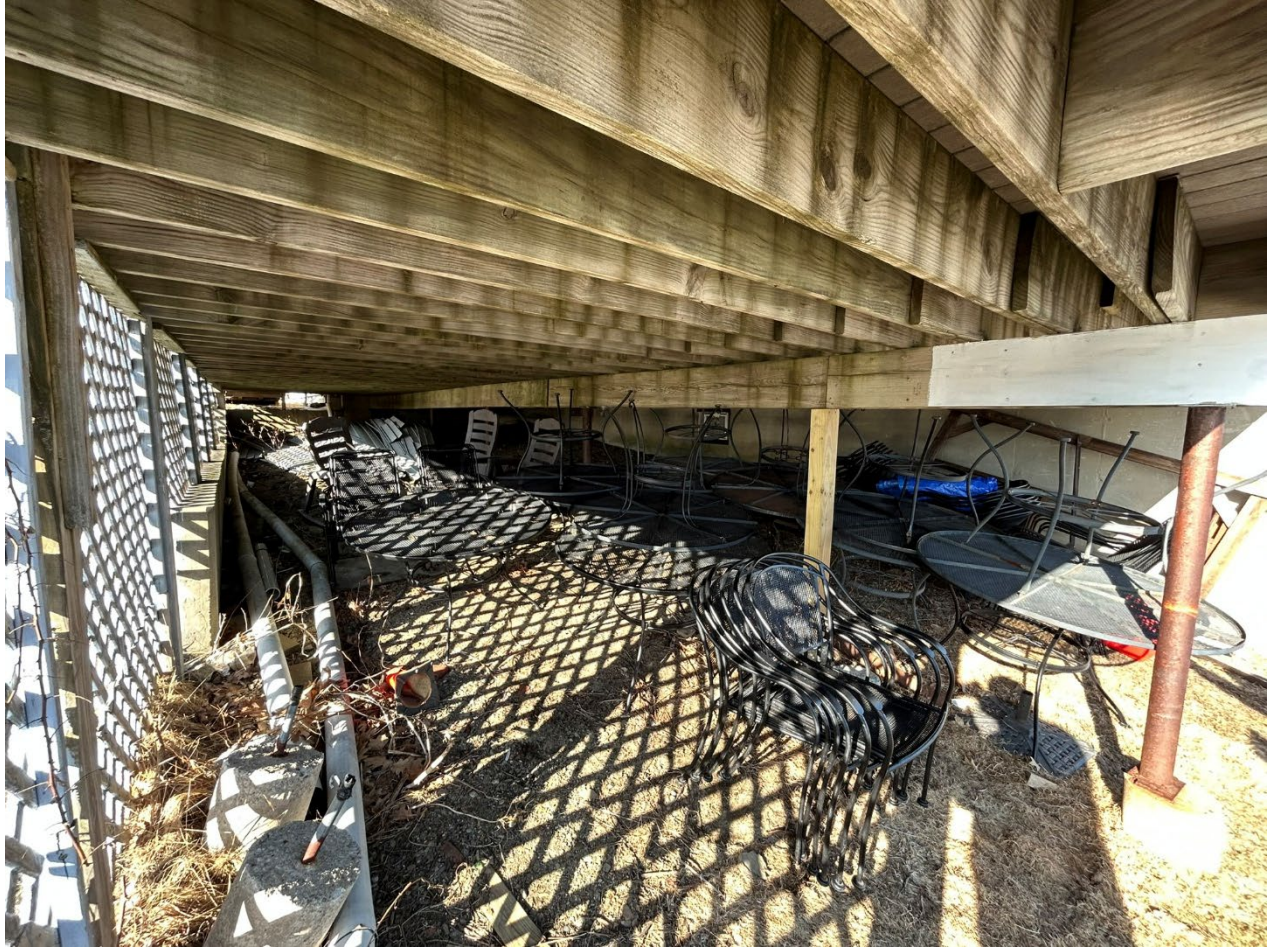
Photo A-2: Underside view of existing deck framing showing aging joists, beams, and limited structural clearance.
