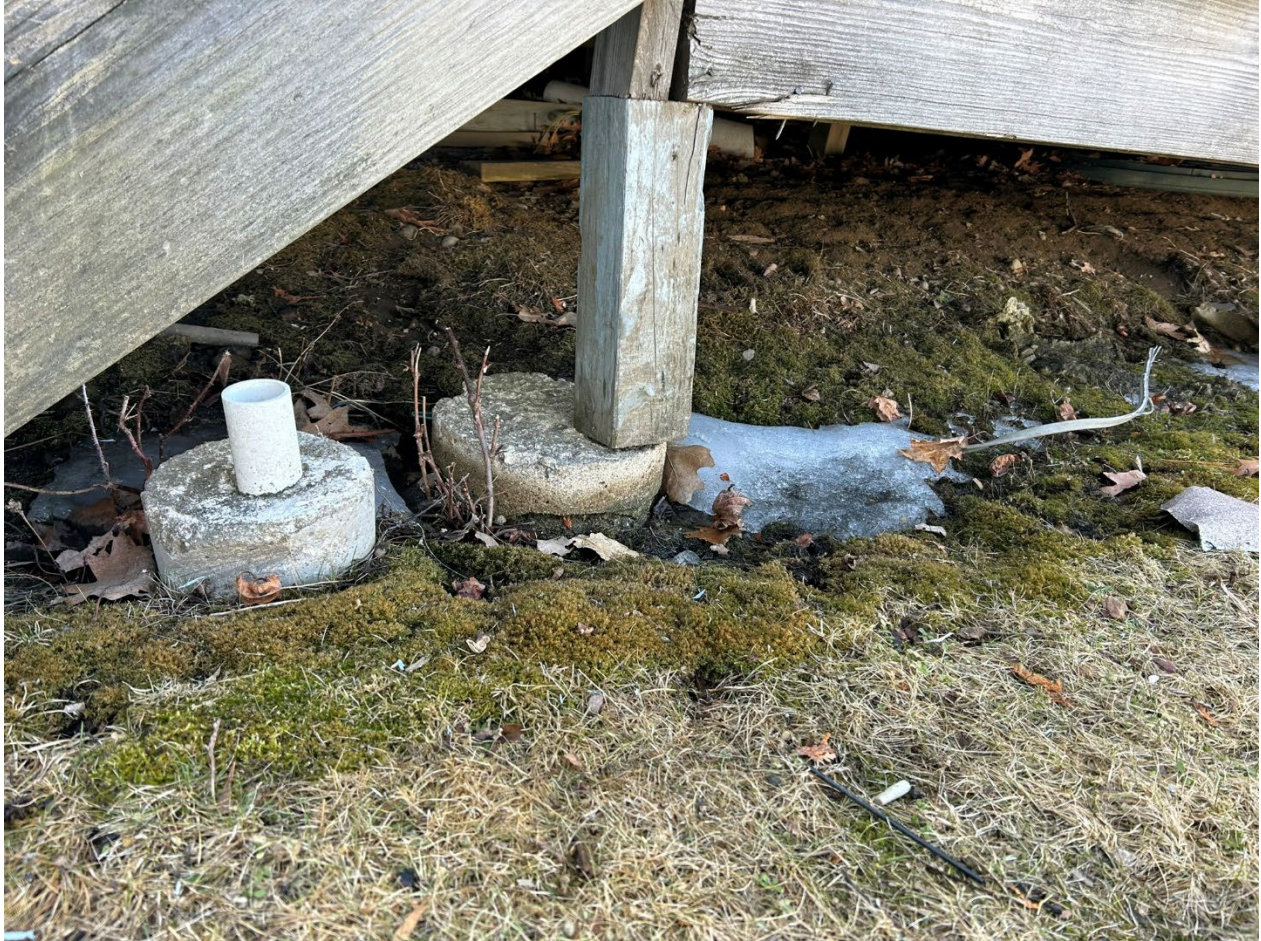
Photo A-7: Close-up of existing pier and bearing conditions illustrating inadequate foundation sizing for current use.
